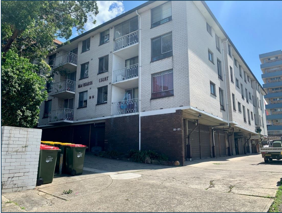
Figure 2 – The existing site comprising of a 3-storey residential flat building above car parking.
